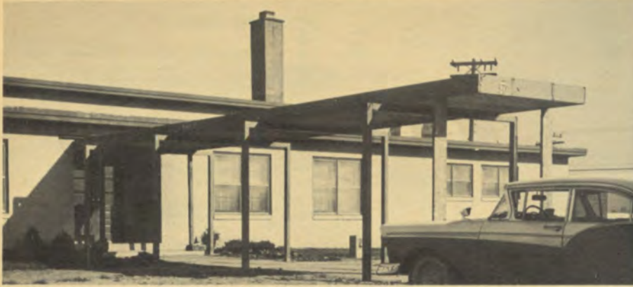
ENTRANCE TO THE NCO OPEN MESS in final stages of completion.
